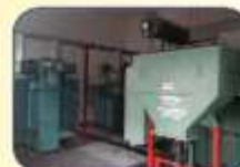
Repairing & Servicing of Transformer up to 5 MVA
